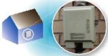
Locate your telephone Network Interface Device (NID). This is usually a grey plastic box on the outside of your home where telephone service enters. It may also be in your basement or garage. This box is a demarcation point between the local phone network, owned by the local phone company, and your home wiring, owned by you.
