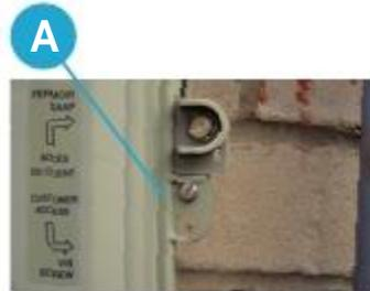
Open the "customer" side of your NID (A). You should see one or more phone lines plugged into phone jacks (B) or one or more sets of wires connected to terminals (C); these are the phone lines coming into your home. If you have one phone line there will be likely be only one connection.
